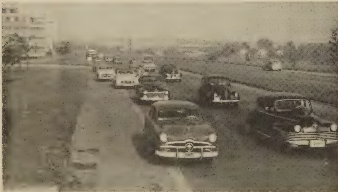
Entrance turn from ramp to freeway. Although traffic from the ramp is rather light, it is sufficient to fill the available spaces in the first lane of the freeway. The lane adjacent to the median is almost devoid of traffic. This characteristic tendency for traffic to distribute itself between lanes results in many of the spaces being shielded against occupancy by vehicles from the ramp.
